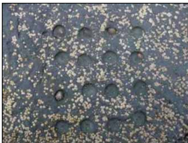
Figure 6: Using artificial niches (holes, 24 x 10 mm) to enhance limpet stocks on a basalt seawall, São Roque, Portugal. (Photo: G. Martins).
