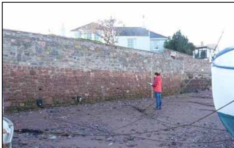
The enhanced wall at Shaldon, Devon. Niche habitat and textured panels were incorporated at the base of the wall.
