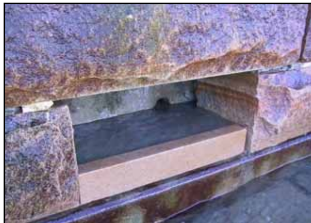
Figure 7: Artificial pools in a vertical sandstone wall, Sydney Harbour, Australia (Photo: G. Chapman, EICC, University of Sydney).
