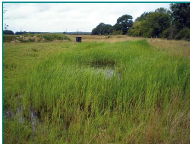
SUDS site, Waterlooville Photo courtesy of Environment Agency
