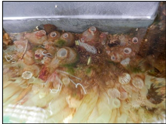
Photos 7 & 8 – Underside of pontoons with growth, Stranraer
