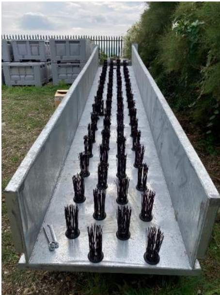
Photograph Ouse 1. The recently installed (Oct-Nov 2023) fish pass on the weir downstream of the survey site.
